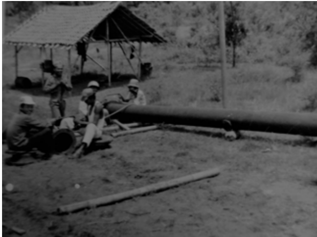
Work on the pipeline, Project Manisrenggo, Indonesia 1973
